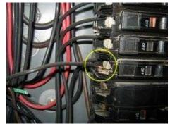
Photo 1 Main service panel-one circuit breaker has a double tap (two wires connected to the same breaker)
