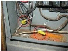
Photo 2 Open splice in the electrical service panel.
