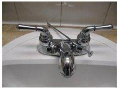
Photo 33 The hall bath sink stopper is not connected.
